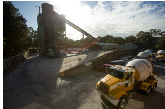
Concrete plant in Alexandria
